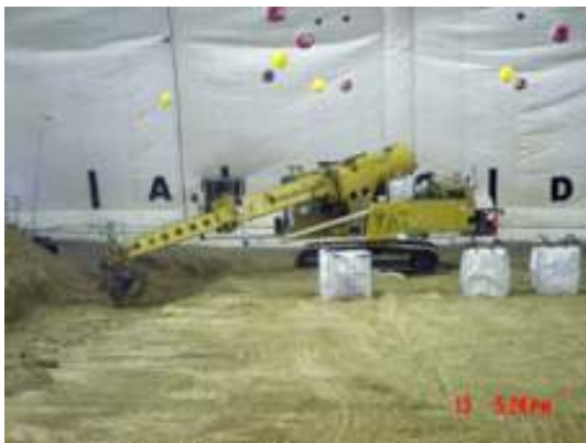
Overburden removal in INEEL's Pit 4.
