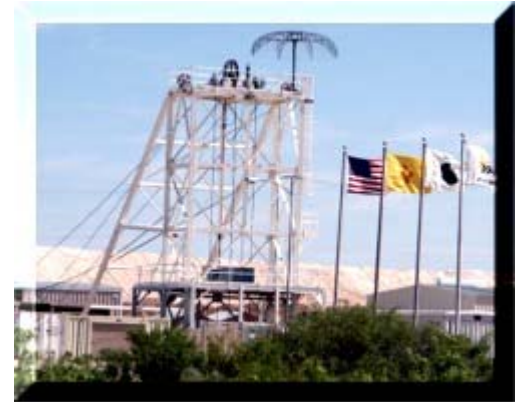
Air Intake Shaft Lightning Protection System
