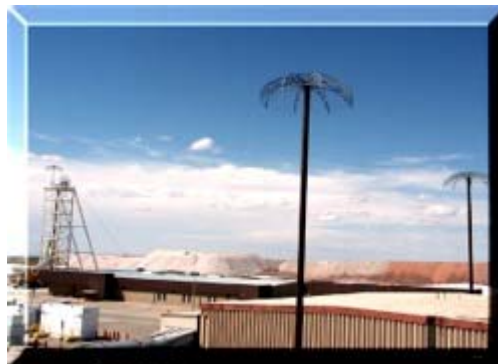
These umbrella-looking devices are part of WIPP's dissipation array.
