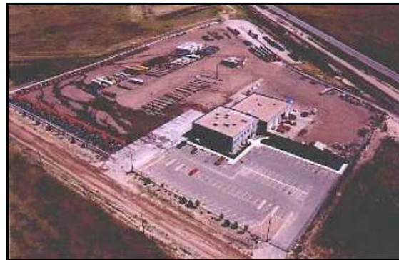
Aerial view of CAST Headquarters
