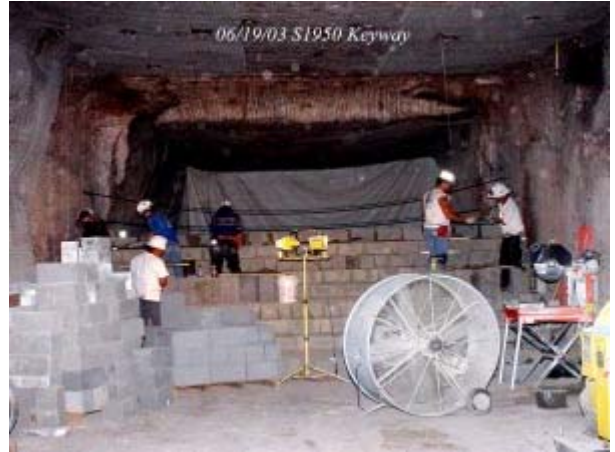
Panel 1 closure wall under construction
