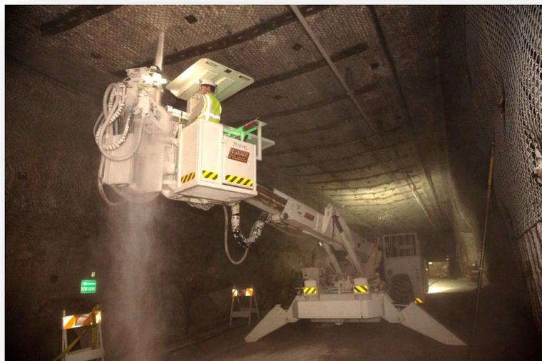
**Ground control activities, like rock bolting, ensure the WIPP underground is safe.**
