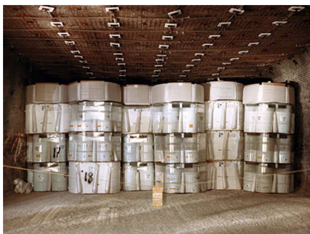
Fig. 2. Actual TRU waste disposed in 55 gallon drum bundles stacked three-high. The MgO sacks are seen placed on top of each TRU waste bundle set.
