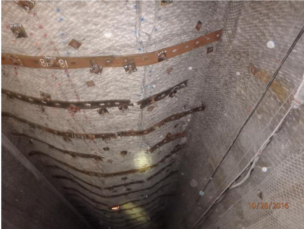
FIGURE 5.—Severe roof bellying in a WIPP drift supported by long tendons, short bolts, straps, and mesh.
