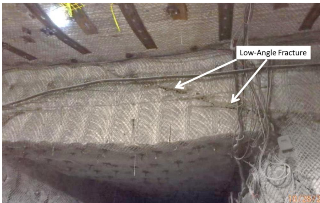
FIGURE 4.—Photograph showing a low-angle fracture exposed in a roof brow.
