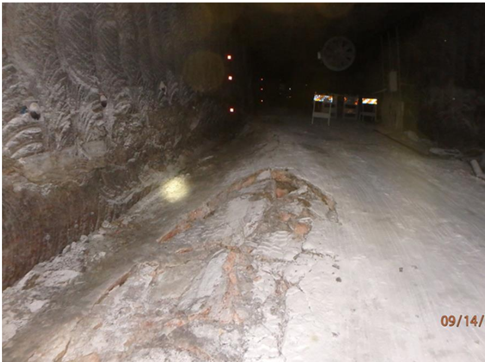
FIGURE 6.—Floor heave in WIPP drift.
