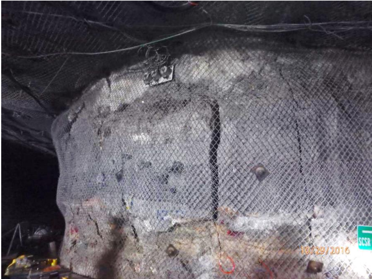
FIGURE 7.—Rib fractures contained by short bolts and mesh.
