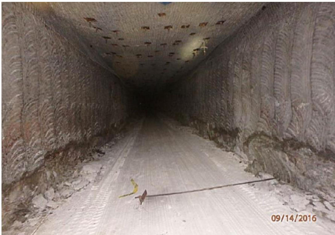
FIGURE 9.—A broken roof bolt that has fallen to floor.
