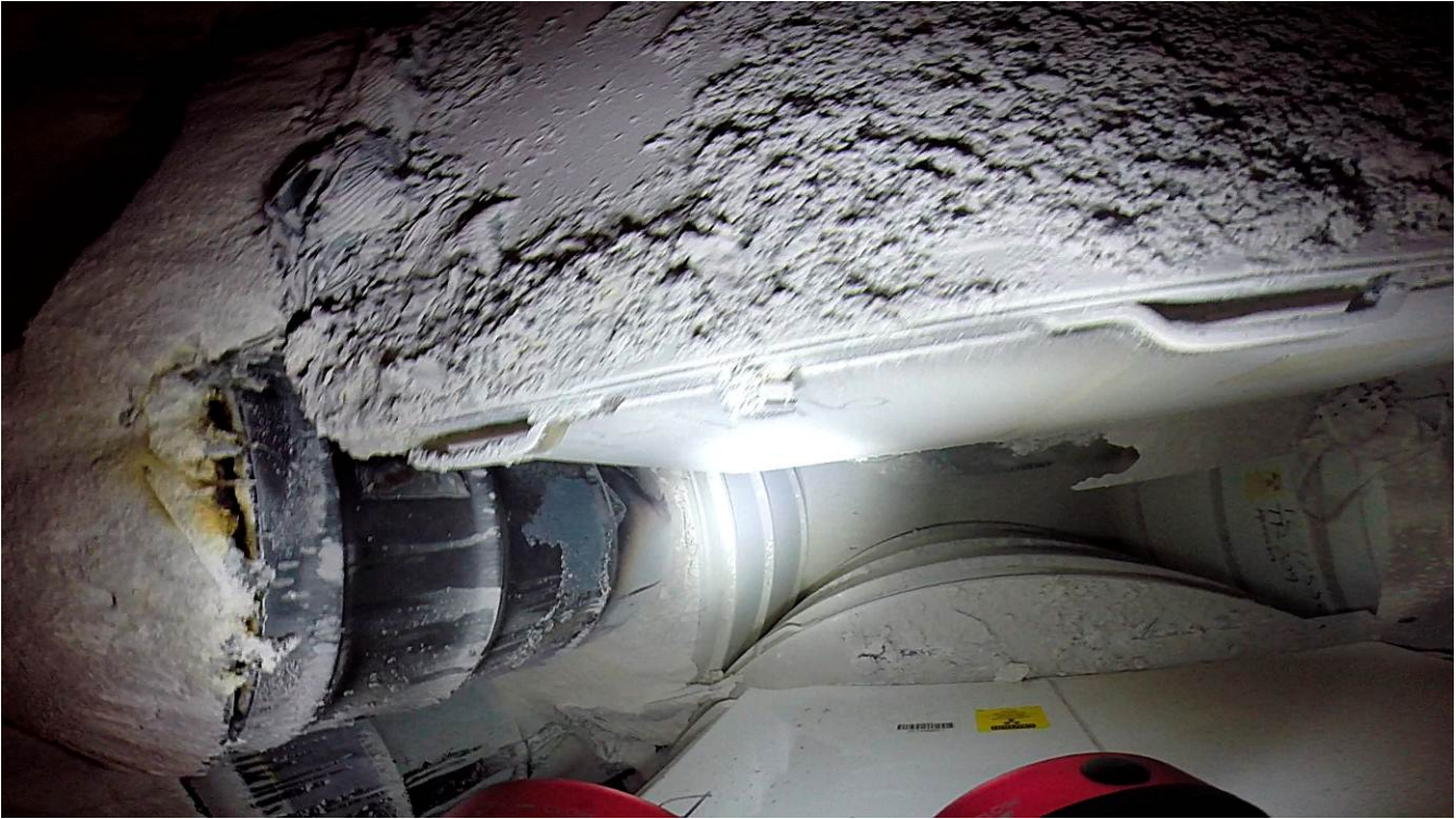
The May 15 entry into Panel 7, Room 7 produced this photo of a waste container (left) with its lid unsealed and apparent heat discoloration.
