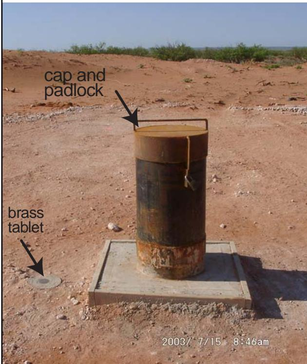
A - Surface casing for SNL-9 with cap and padlock. View to south.
