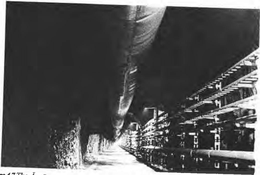
Figure 4.7 The Åspö access tunnel from 205 m and downwards. The height and width are 5.5 m x 5.5 m respectively and the inclination is 7 %. The large tube under the tunnel roof is the ventilation. The picture was taken the 17 of August 1993.
