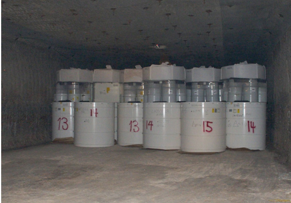
Figure MgO-1. Supersacks of MgO Emplaced on Top of the Waste Stack
