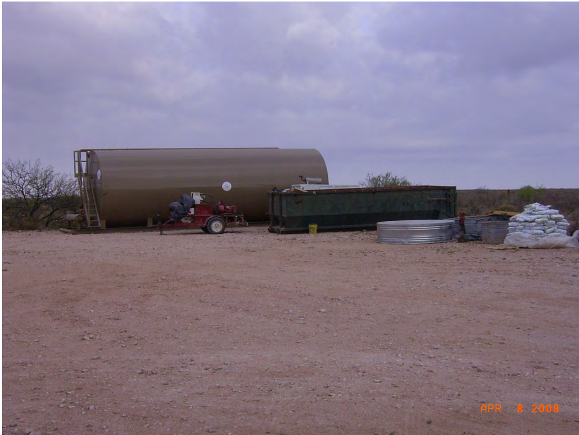
Figure 13 - Dedicated Fresh Water Tank at the Staging Area
