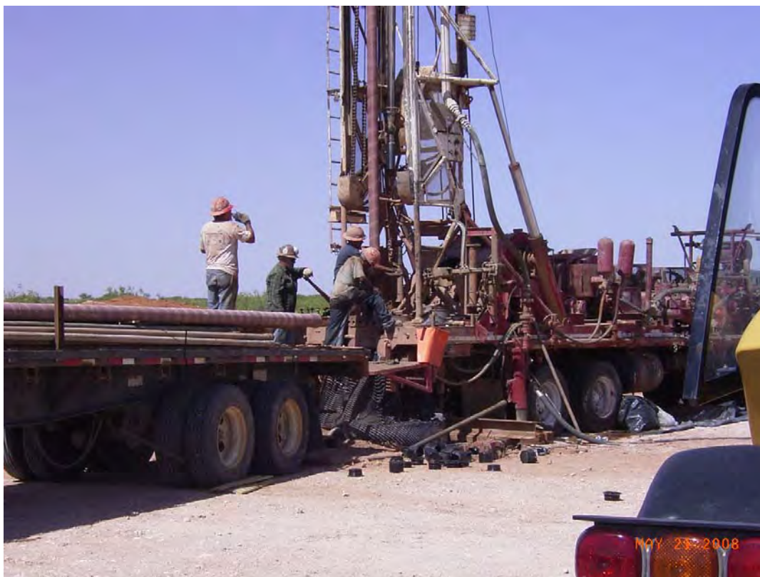
Figure 9 - Setting 5.5-Inch Fiberglass Casing at H-15R
