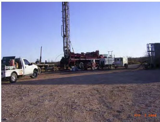
Figure 12 - Air Lift Well Development at H-15
