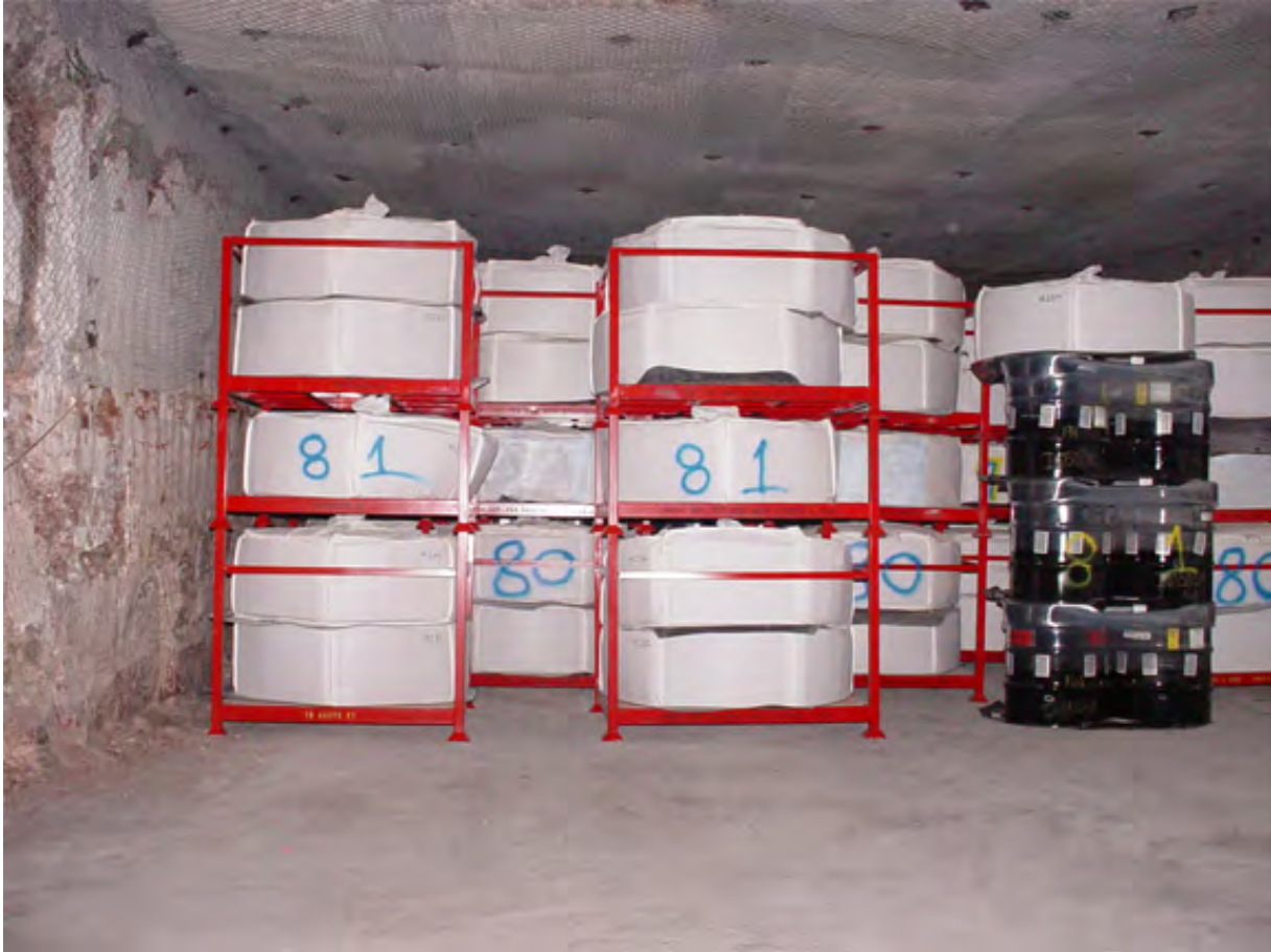
Figure MgO-2. Racks Used to Emplace Additional MgO
