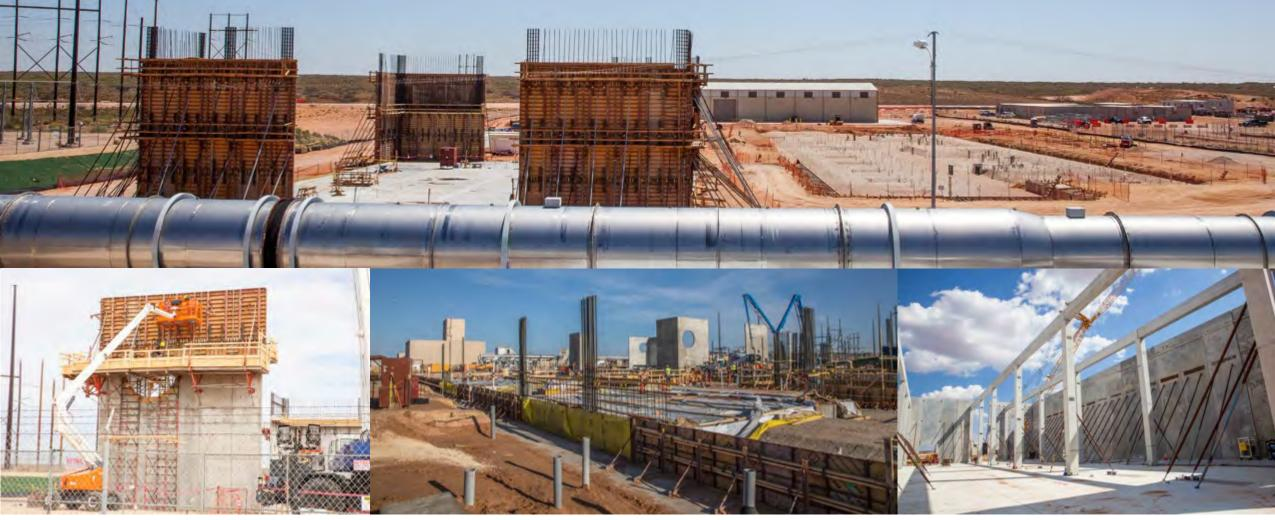
SSCVS overview, showing the concrete walls and rebar of the New Filter building and the roofed in Salt Reduction Building (Right) – November 2021
